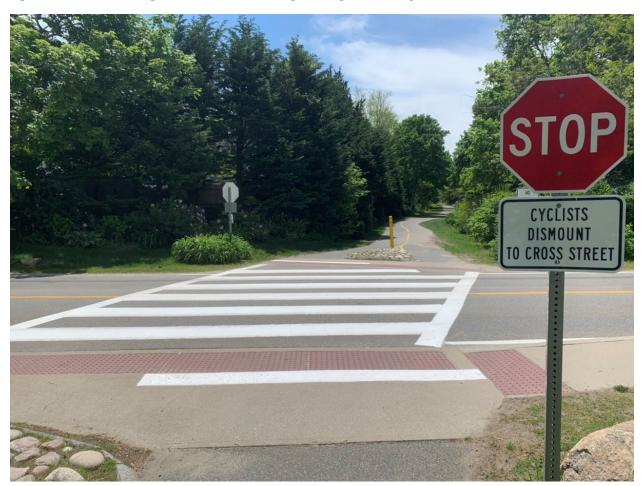
Figure 20: Tactile Warning Plates at a Road Crossing, Shining Sea Bikeway in Falmouth
