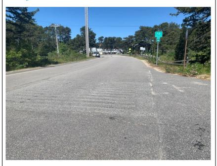
Figure 66: Faded Paint is Used on the Crosswalk. Note the RRFBs.
