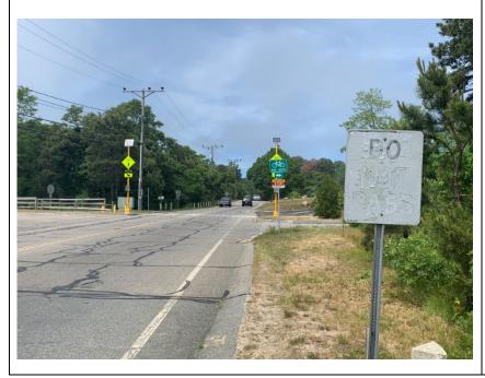
Figure 177: Trail Crossing is STOP Controlled. Facing SB, There is Only a Single RRFB.
