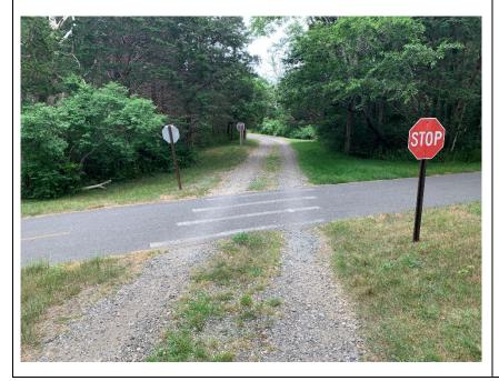
Figure 92: Path Approach. Note the Faded Crosswalk Covered by Dirt from Passing Cars.
