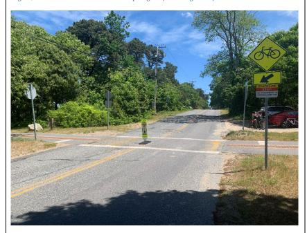
Figure 78: Path Approach. Note the Splitters on the Approach
