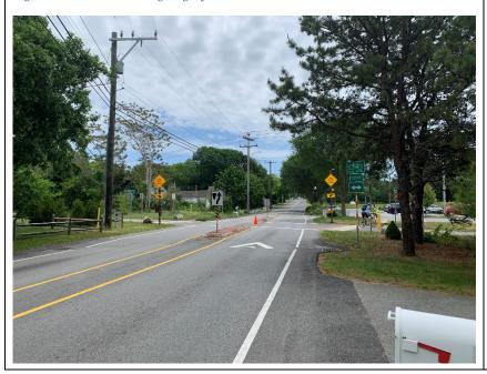
Figure 199: East-Facing View of Path Crossing. Medians Provide a Place for Bicyclists and Pedestrians to Make 2-Stage Crossings
