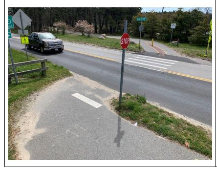
Figure 193: Road Approach from East Side Showing the Bike Trail Crossing Signage and the Wayfinding Signage (Advance Signage is Not in Picture)
