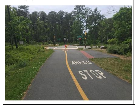
Figure 203: Raised Crosswalk Ahead Signage, Along with Sharrows Demonstrating Bicyclist Crossings
